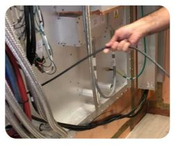
Pull the 40ft cable from another side of the RF closet and connect it to the back
