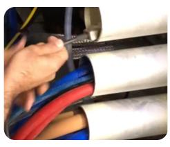
2. Push the 40ft cable into the waveguide.
