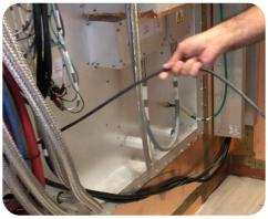
Pull the 40ft cable from another side of the RF closet and connect it to the back of the actuator.
